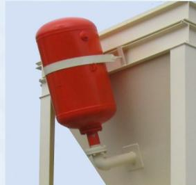
Air cannon mounted on hopper for sticky material.
