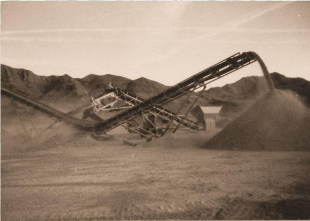
*For over 25 years the Fab Tec Pro Screen has been proving itself in the field with production rates up to 240 TPH producing 3/4" minus.*
